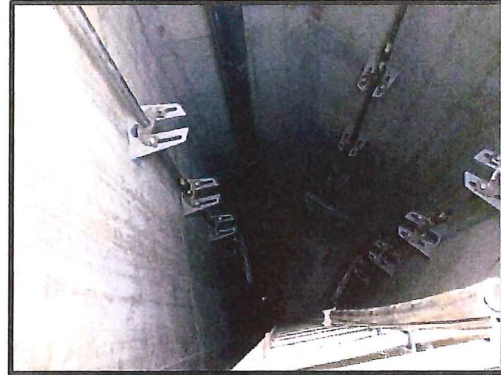
Inside the Completed Junction Structure
