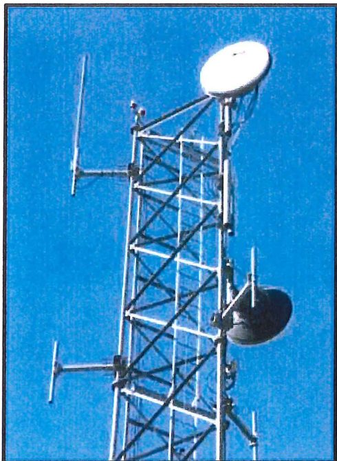
Basin Communication Tower
