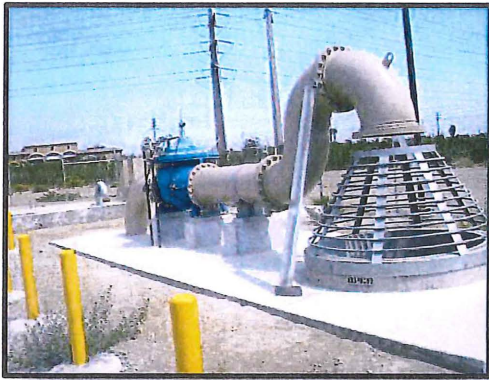
CB-20 Turnout Facility
