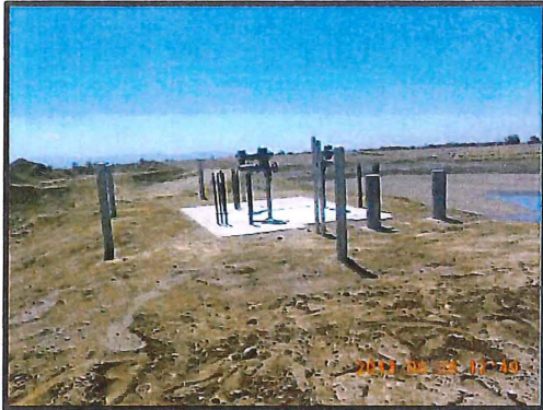
Construction of Junction Structure
