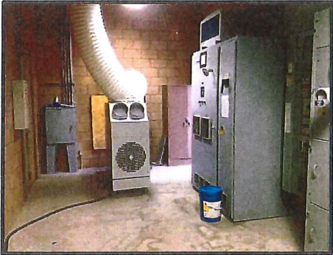
MCC Control Panel
